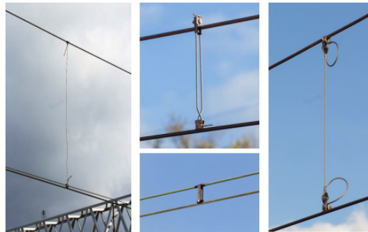
Figure 205: Dropper types (clockwise from left): non-current carrying; chopsticks uplift; current carrying; loop uplift
